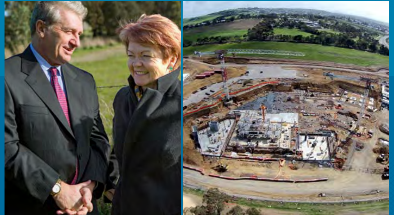
Left. Epworth HealthCare Group Chief Executive Alan Kinkade and Vice-Chancellor, Deakin University Professor Jane den Hollander. Right. An aerial view of construction at the Epworth Geelong site
